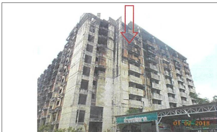
1st high building, 11 storey
